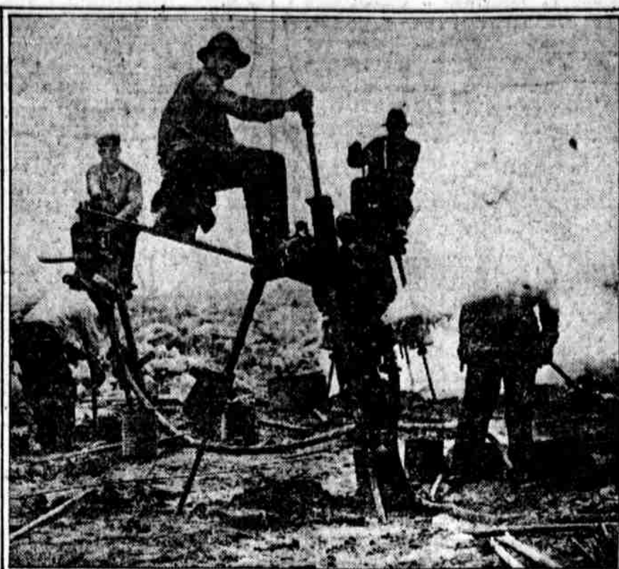
CITY IMPROVEMENT. The task of moving a large hill from the edge of Fairmount Park, at the Green street entrance, and the building of the Art Gallery is progressing nicely. Three drilling machines were found in action as they bored into the rocks that will be removed. Then, on another section of the site, steel workers were riding girders to their places. Ledger Photo Service
