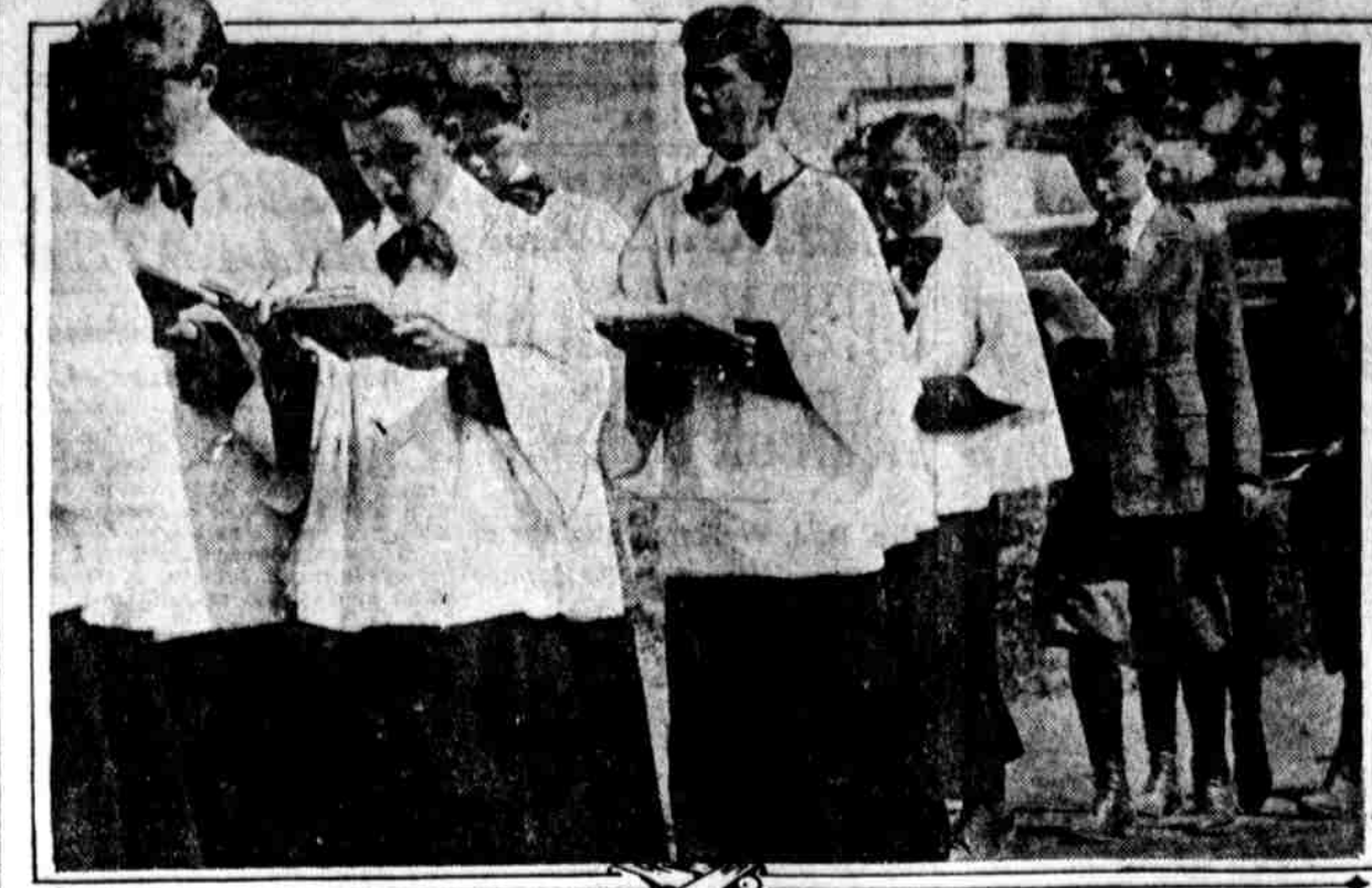
Yesterday afternoon ground was broken for the new Administration Building of the Church Farm School at Glen Loch, which is conducted by the Protestant Episcopal Church. Three cottages were also dedicated. In all these ceremonies the Right Rev. Philip M. Rhineland was in charge.
