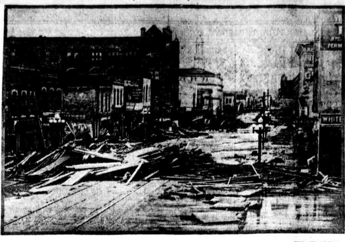
First photograph of one of the business streets in Pueblo after the floods had begun to recede. Waters from the outlying districts swept through this avenue, leaving it almost choked with wreckage. The large building in the background is the courthouse.
