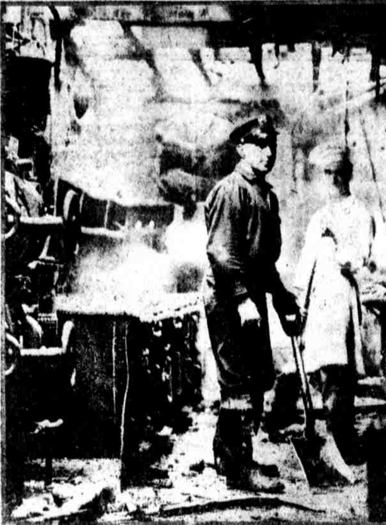
Thommen's restaurant kitchen, market street above Fifteenth, in ruins. The picture shows the chef getting breakfast under difficulties.
