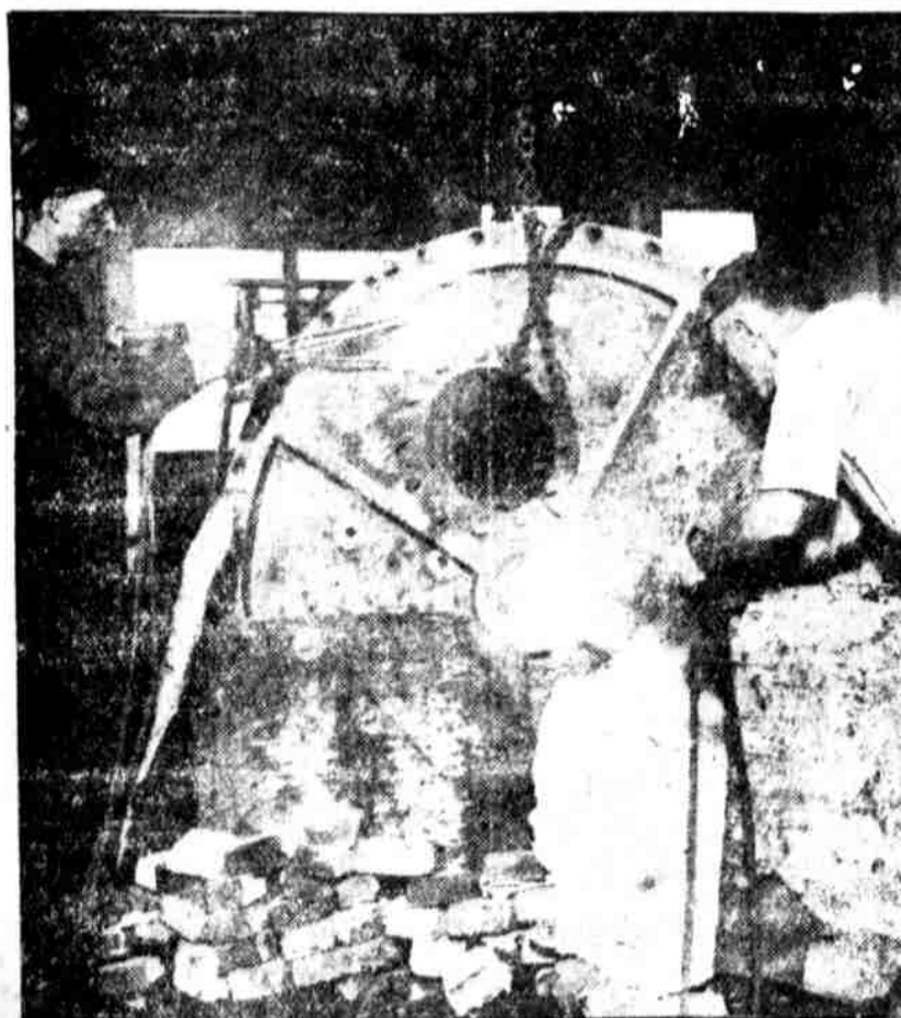
RUBIN SCHWARTZ AND L. D. HANDY welding a condenser head of a ship at the National Electric Welding Company, 6 North Twentieth street. Ledger Photo Service.
