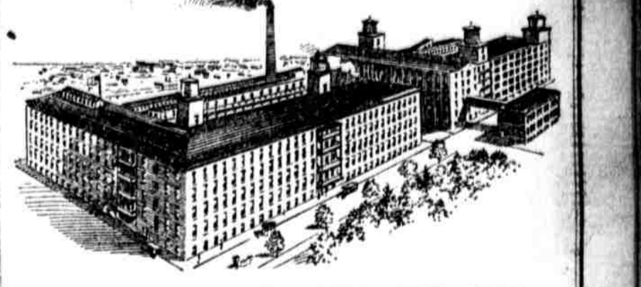
LARGE KENSINGTON MILLS FOR SALE 250,000 square feet ground area, 500,000 square feet floor area; the best large, modern, modern manufacturing plant, with railroad siding, for sale in Philadelphia; will sell individual units. For particulars apply to:
