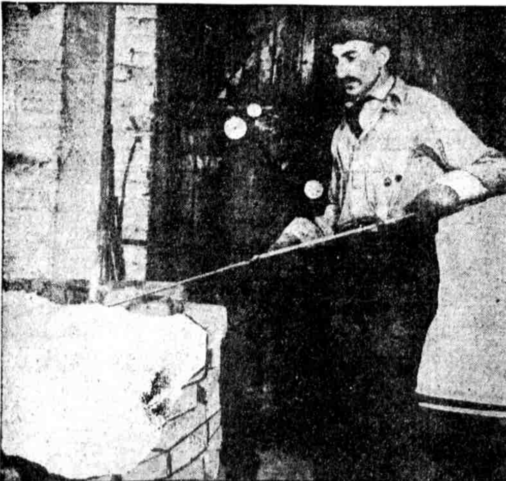
BENJAMIN HEYMAN handling a welding machine at his shop, Hunting Park avenue and Fox street. The welding is done by gas
