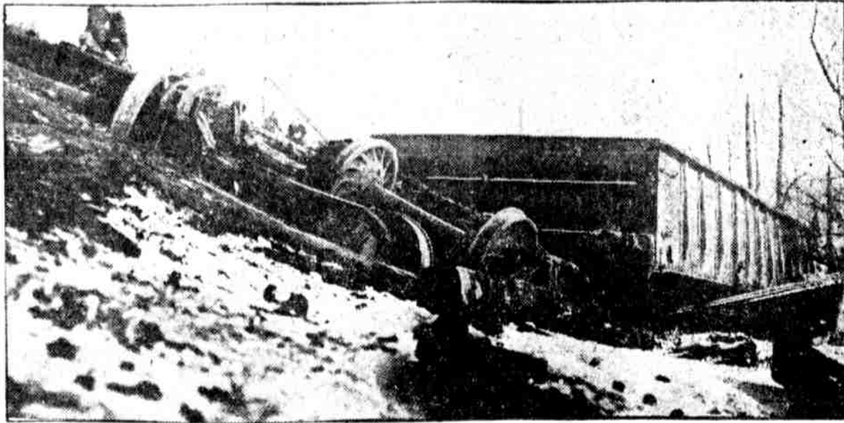
A PART OF THE PENNSYLVANIA RAILROAD SPILL. While five tracks were covered with wreckage at Plainsboro, N. J., most of yesterday, some of the wrecked cars went over the embankment. It will take several days to clear up the debris.
