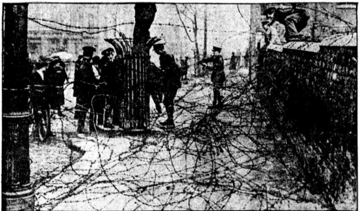
PROTECTING DUBLIN CITY HALL. This wire entanglement is being erected preparatory to the occupying of the city buildings by the British soldiers. They will do guard duty. Underwood & Underwood.
