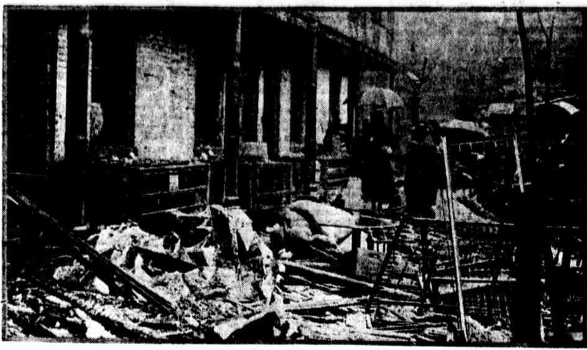
The picture shows what was left of homes back of the stable at 506-516 New Market street after they had been attacked by flames spreading from a fire that destroyed the stable. The household goods the tenants were able to remove are seen. The fire occurred last night and was discovered shortly after a man who had bought some matches was seen entering the stable.
