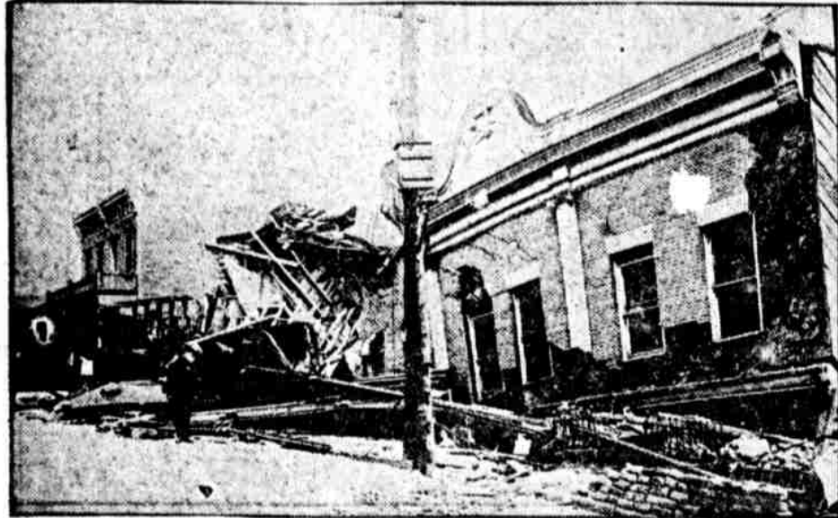
DAMAGED HOUSES IN SCRANTON. The sinking earth, due to mine caves, continues to wreck property in the Lackawanna county city.
