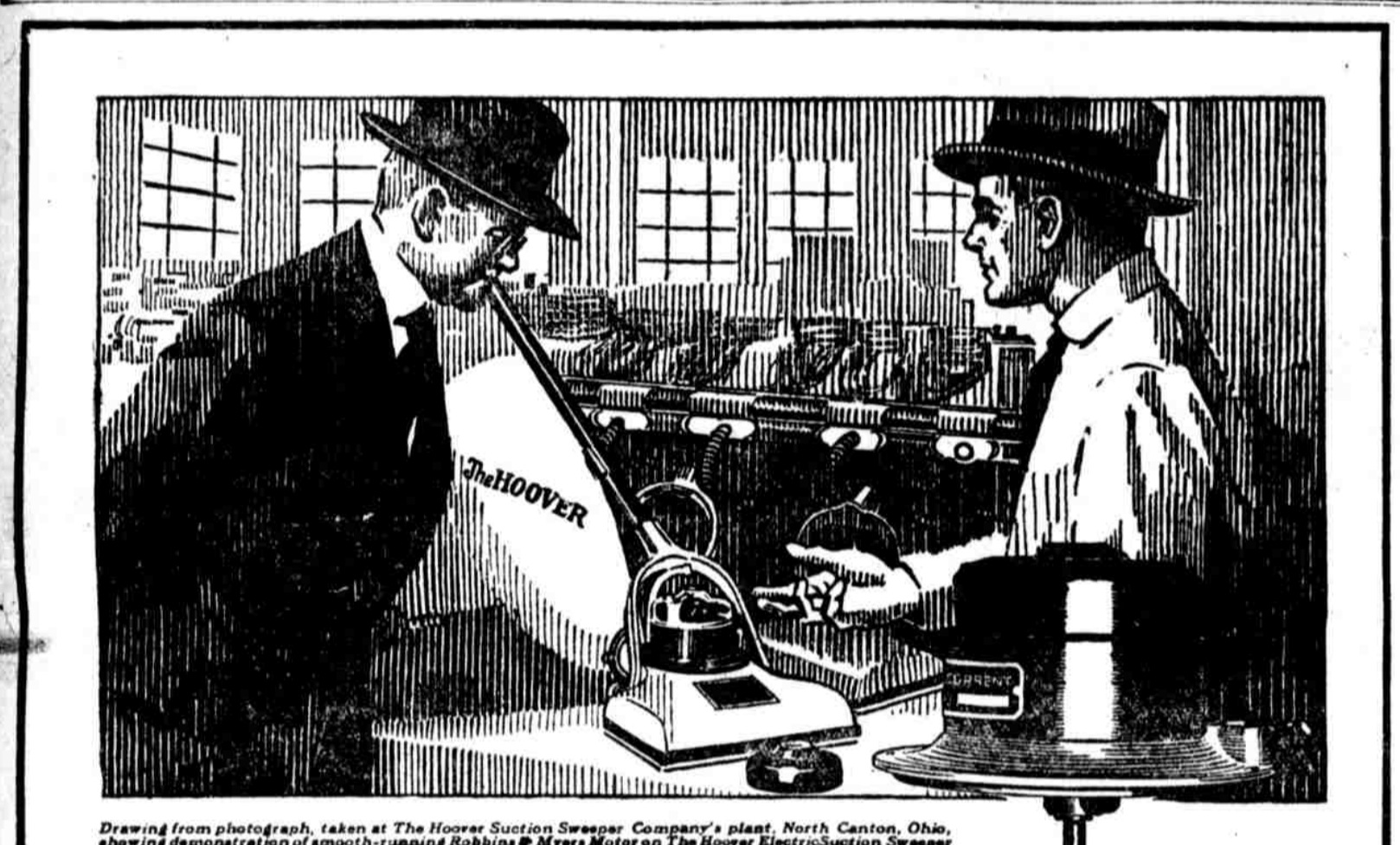
Drawing from photograph, taken at The Hoover Suction Sweeper Company's plant, North Canton, Ohio, showing demonstration of smooth-running Robbins & Myers Motor on The Hoover Electric Suction Sweeper
