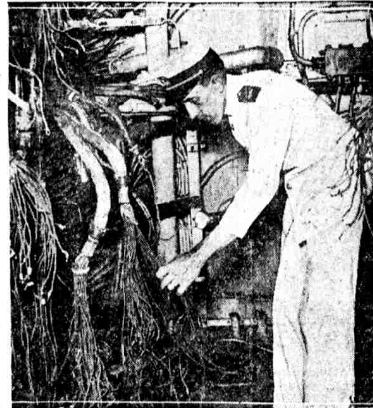
THE CONDITION OF GERMAN SHIPS when turned over. Former German warship Ostfriesland was found with instruments smashed, wires cut and everything ripped apart when taken over by Americans. Gunner F. C. Struss is making an examination. Kadel & Herbert.
