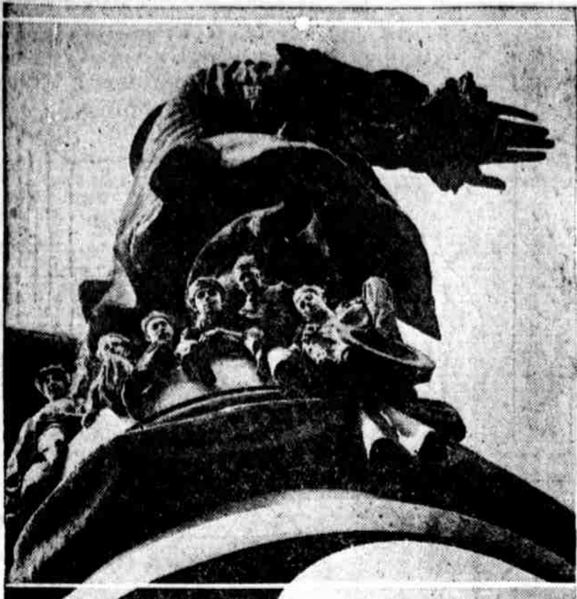
BILLY PENN, WHO HAS A STATIONARY POSITION on top of City Hall, is being repainted, repaired and made to look his best. An Evening Public Ledger photographer yesterday snapped the 'sleeplejacks' as they rested at Bill's right foot. Ledger Photo Service.
