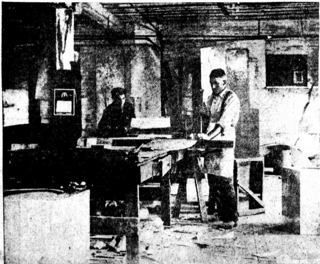
SAMUEL GREENSPAN, 3838 Folsom street, rolling tops for pipeless heaters (left), and Bert Henderson riveting the cone tops at the Frederick S. Sabin Co., 237 Broad street.
