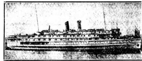
The NOPATIN (ex-MANHATTAN) and NARRAGANSETT are sister ships. built in 1913. They are 3.539-ton steel ships, with passenger accommodations for about 532. Length 320 feet, breadth 48 feet 1 inch, draft 16 feet. Cargo space between decks approximately 45,000 cubic feet. These vessels have a recorded speed of 23 knots and are ideally suited for Sound, river or coastwise service. They are excellent seagoing vessels and during the war carried troops across the ocean.
