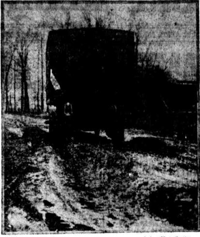
Deep mud holes, a succession of long ruts, together with large piles of dirt, make up a section of the Lincoln Highway in the confines of the state of Pennsylvania. The photograph was snapped at Morrisville, Pa., which is across the Delaware river from Trenton
