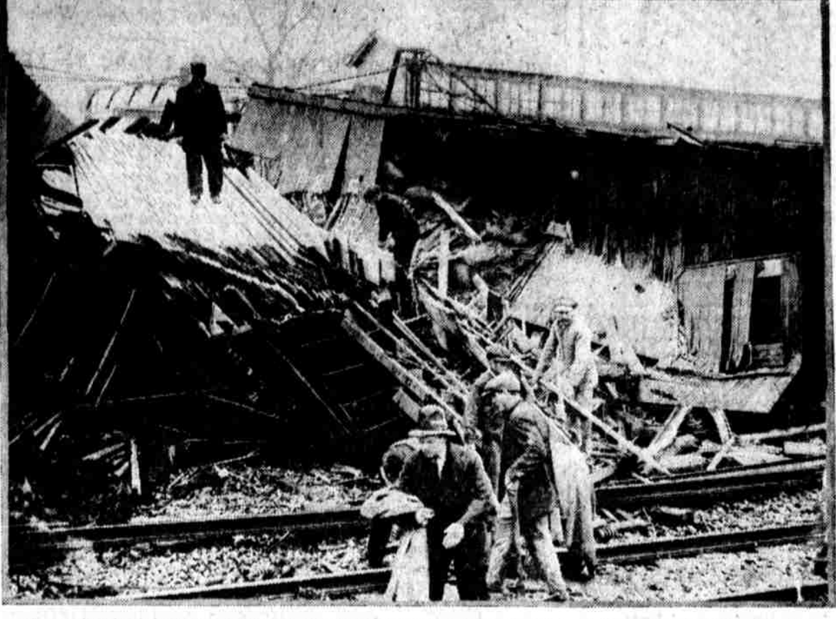
Great pile of debris which blocked all four tracks of the Pennsylvania system at St. Davids for eight hours this morning.
