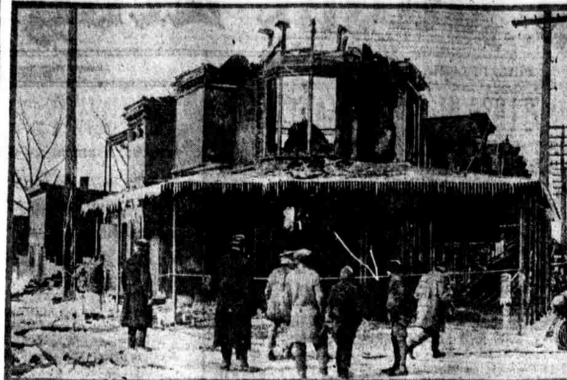
Only the walls remained after the devastation the department store of Sichelroth Bros., 4632-40 Lancaster avenue, at 2 o'clock this morning.
