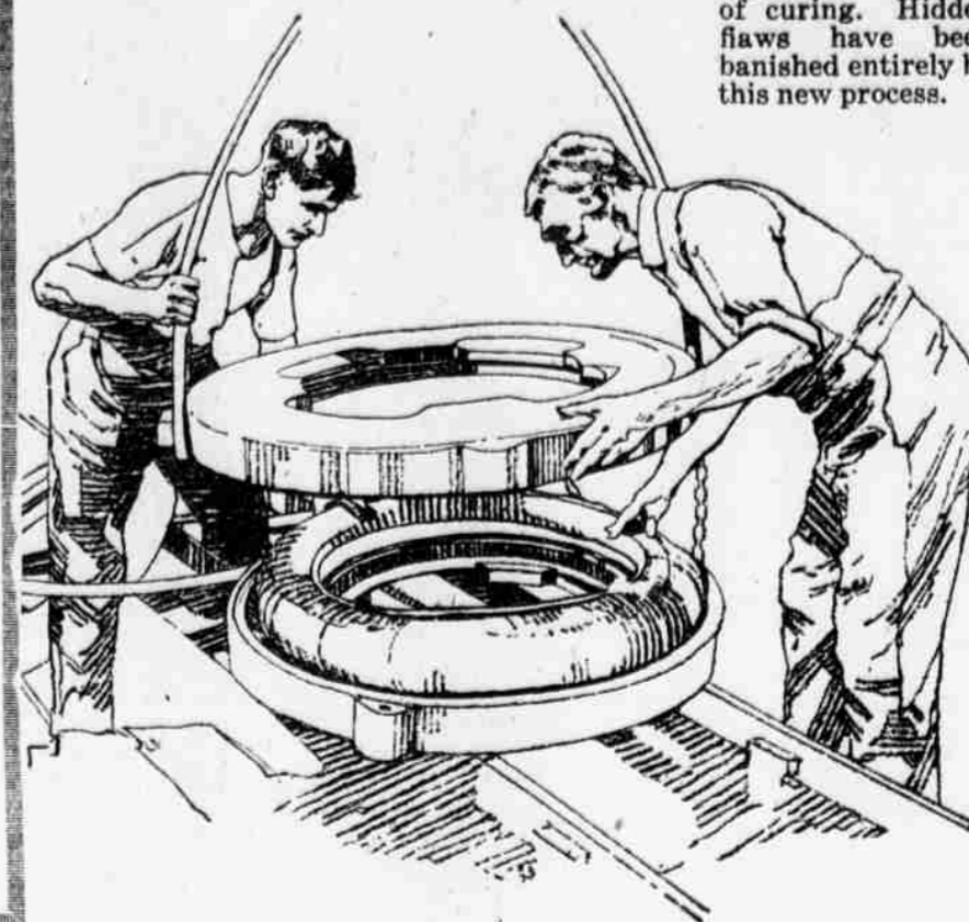
Curing by internal pressure insures a structurally perfect tire.
