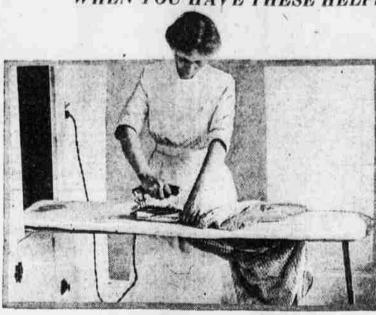
The ironing board is fastened to the wall with a hinge that allows it to be folded up out of the way when not in use. A brace is also hinged on the board, and may be made long enough to reach back to the wall, or merely long enough to reach the floor like a table leg. If you have this kind of a board and the electric iron that the housewife in the picture is using, what's to prevent your cheating the laundry out of a half the usual bill by doing some of your ironing at home
