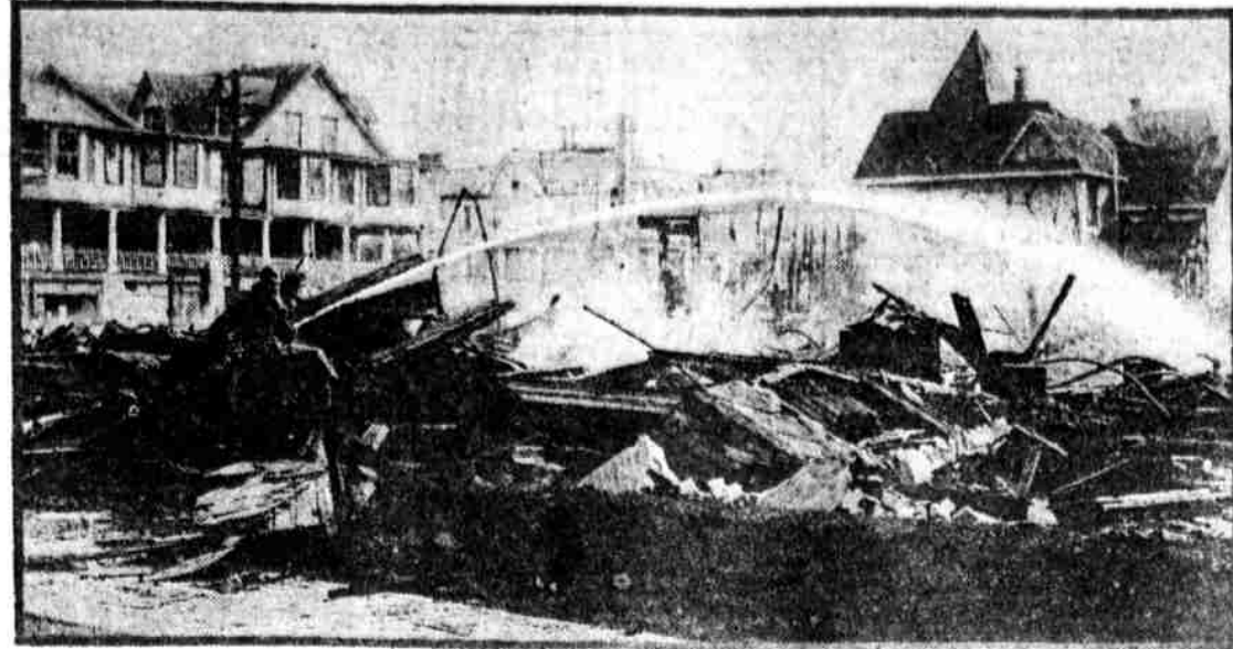
The fire in Wildwood, N. J., of undetermined origin, destroyed the Coombs Building and the home of Francis W. Devlin, besides damaging the Marine National Bank, the Seacrest Hotel, Caldwell Building, Varsity, Cedarcroft Apartments, Plaza Annex and many stores and business places on the street floors of the buildings. The fire ruts in the view are directly opposite the Coombs Building, looking south on Pacific avenue.
