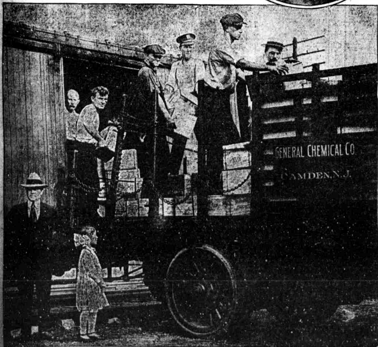
Photo by LEDGER PHOTO SERVICE
