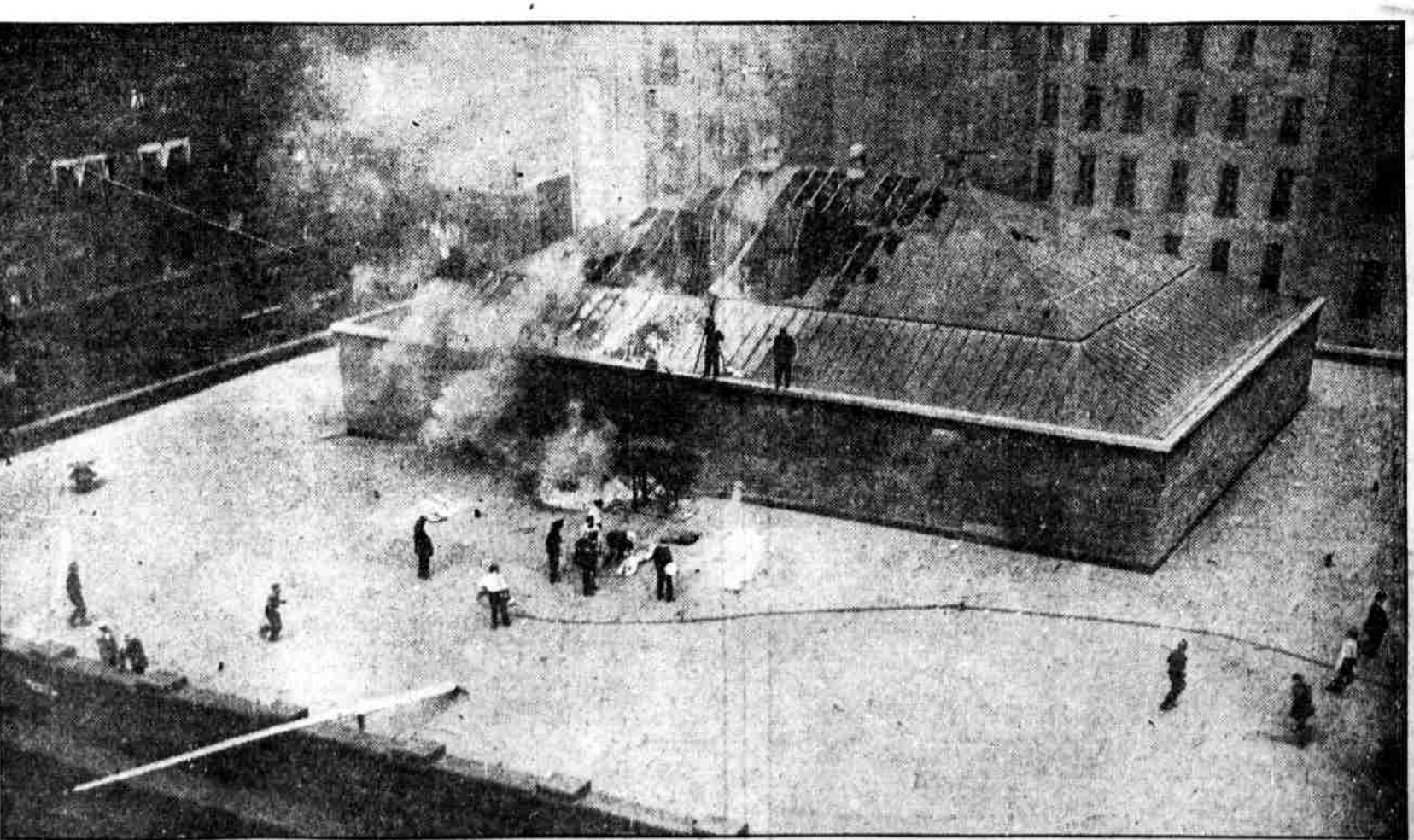
THE SHATTERED SKYLIGHT, through which the blazing dirigible crashed into the Illinois Trust and Savings Bank, showing firemen at work on the roof
