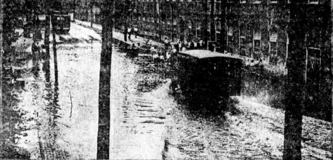
A sewer, choked by heavy rains, was responsible for eighteen inches of water in the delirious between Wissahickon hill and Walnut lane, on Main street, Manayunk, blocking traffic and flooding the basements of nearby mills.
