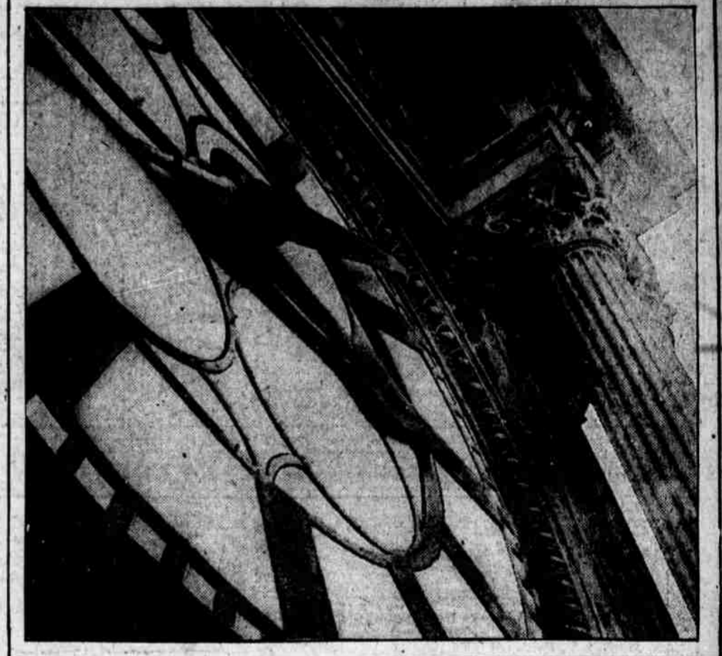
AN AWRY VIEW of Philadelphia's chief timepiece from a tower ledge beneath the great dial. The minute hand is 10 feet 8 inches in length and weighs 225 pounds. The hour hand is 9 feet long, weighing 175 pounds. The minute hand travels 114.7 miles in one year.
