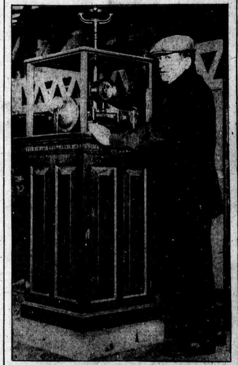
THE AIRTIGHT and dustproof case inclosing the master clock that operates William Penn's great timepiece. Once every minute the clock opens the valve which admits compressed air to the tubes connected with the gears operating the huge hands of the great dials.
