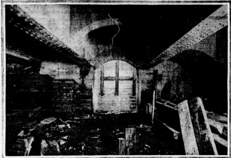
entrance stairway leading from the southwest corner of the City Hall courtyard into the subway. The entrance has been cut through the foundation Through the most skillful engineering work it has been possible in building the new subway to underpin the foundations of the building with concrete and girders and pillars of steel, insuring complete stability and security to the great structure overhead
