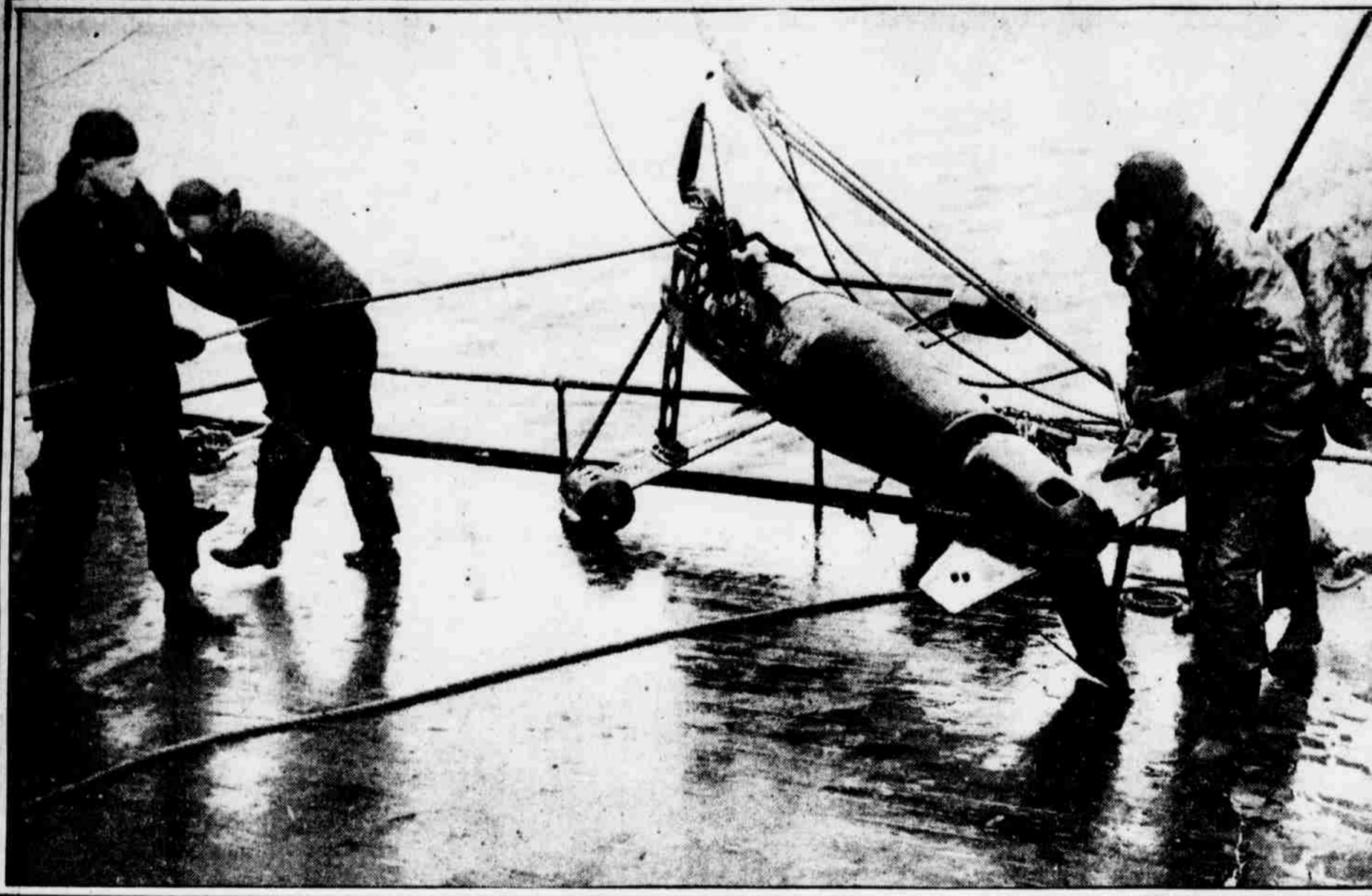
THE PARAVANE, A BRITISH NAVAL DEVICE to destroy mines, adopted by the American navy. It is a torpedo-shaped construction, with fins at its head and a rudder contrived to keep it at any depth. A wire rope, by which it is connected with the ship, catches up the mooring ropes of the mines and causes them to travel to the nose of the paravane, where a sharp saw severs them. The mines, set free, may be seen and destroyed.
