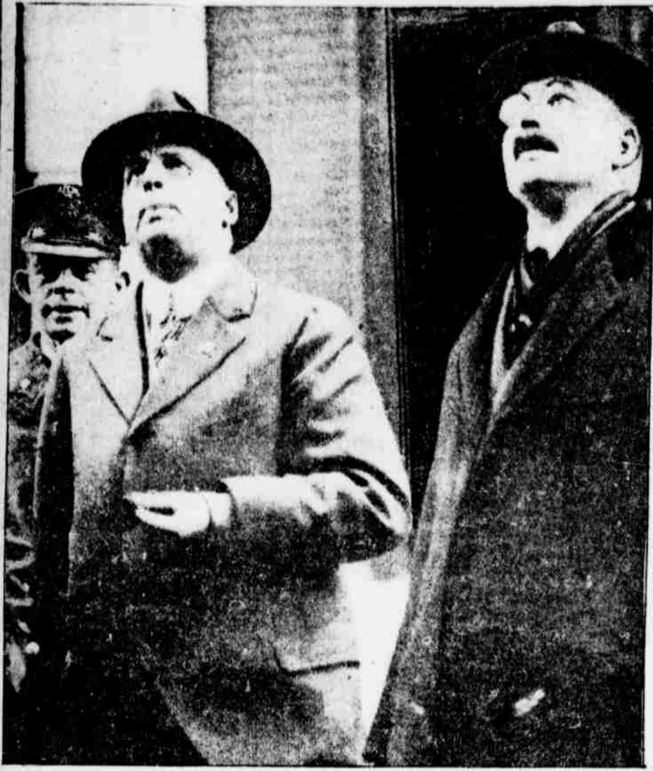
JUDGE WILLIAM GRAY KNOWLES, of the Municipal Court (at left), viewing the damage done to his home, 2102 De Lancey street, by the bomb explosion on Monday night.
