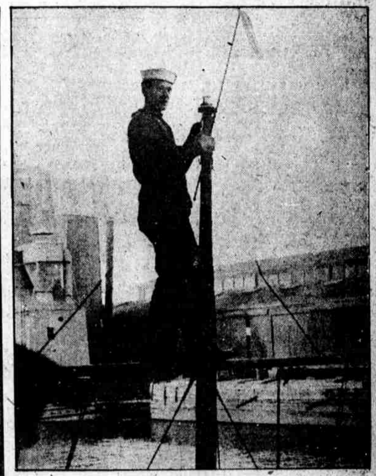
REMOVING SIGNAL LAMPS
