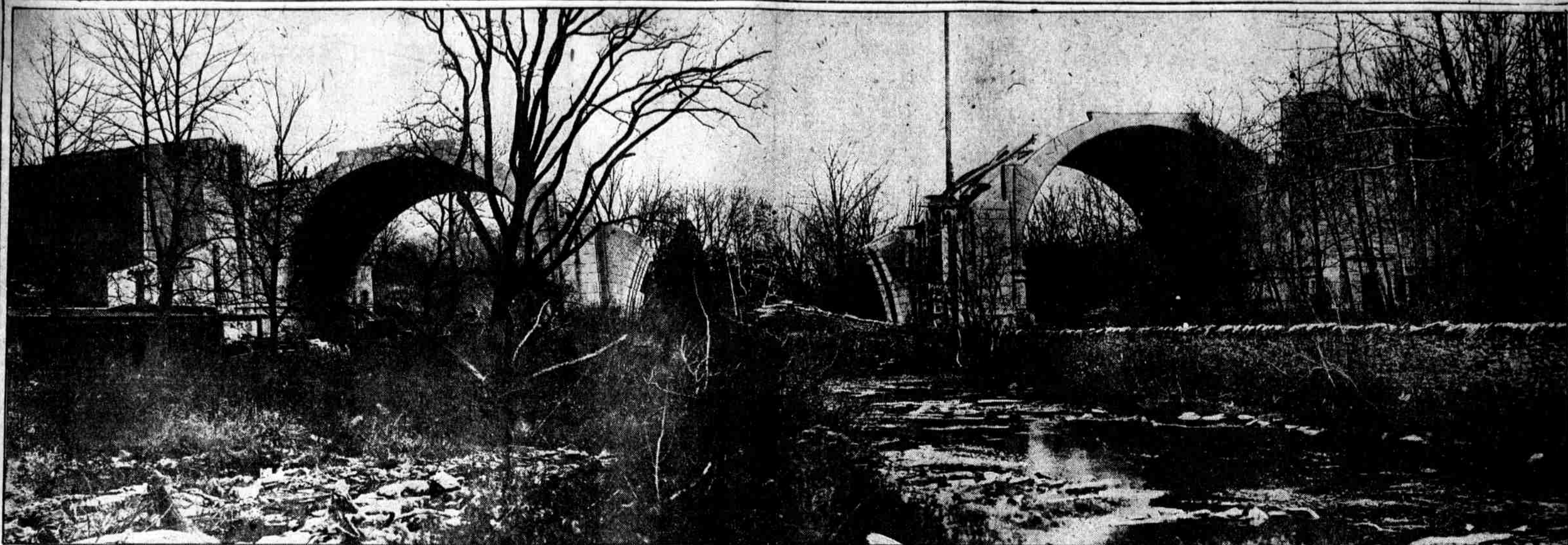
BENSALEM BRIDGE construction, at the end of the Northeast Boulevard, was delayed during the war by the shortage of labor and material. The release of hundreds of workers from the war industries and the removal of the city work ban will permit, it is hoped, an early completion of the bridge
