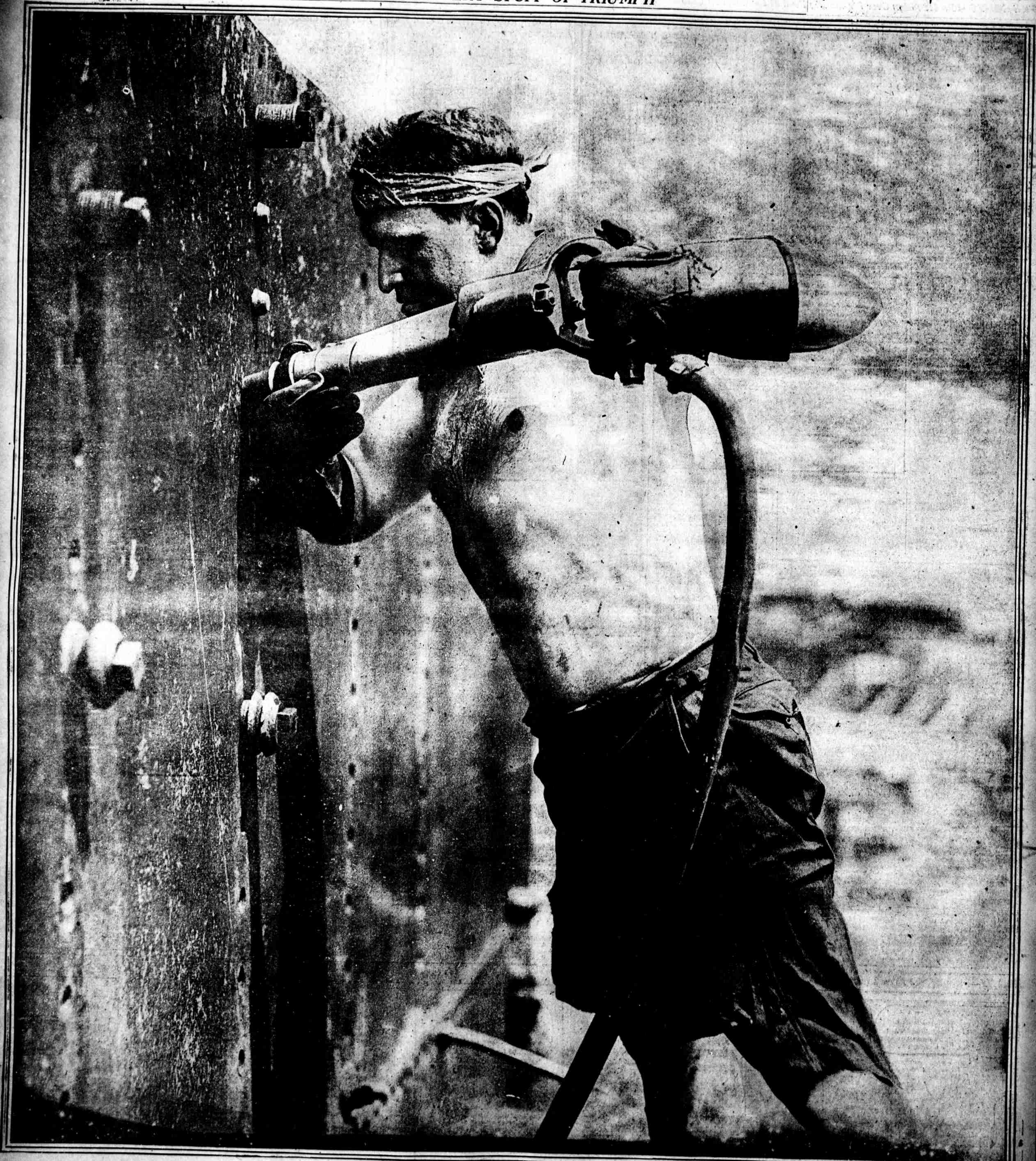
THE AMERICAN SHIPWORKER DEFIES RECORD-MAKING HEAT IN HIS HEROIC FIGHT FOR FREEDOM "The Spirit of '76" animates this Hog Island riveter, who, under a blazing sun that radiated blistering heat from the steel hull at which he and his companions worked, drove bolt after bolt home that no time might be lost in America's shipbuilding schedule.
