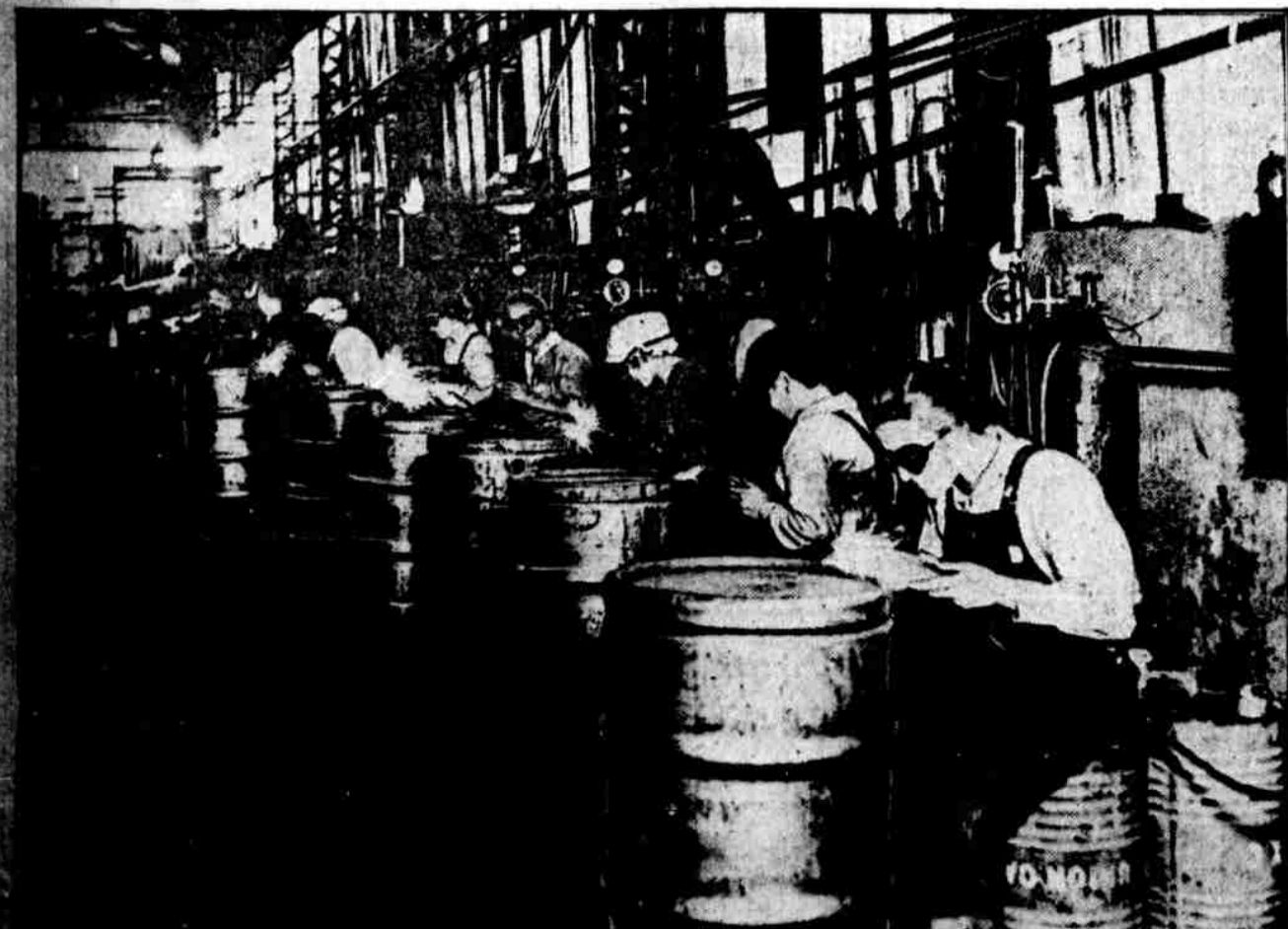
OF COURSE, THE WOMEN WELDERS employed in a California steel works are making good in this realm of molten iron and flaming torches.
