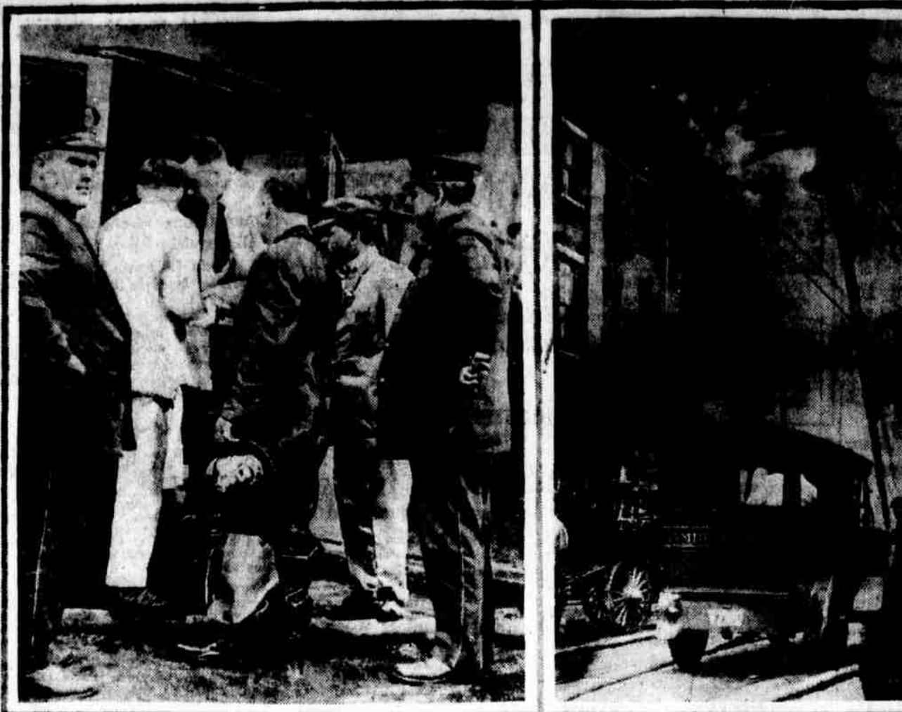
Flames spread rapidly when an exploding gasoline tank let loose in the garage to the rear of Louis E. Wiser's furniture factory and warehouse at 260-262 South Fifth street, and soon the four-story structure was a roaring furnace. Three firemen were injured fighting the blaze, one of the photographs above showing an injured man being taken into an ambulance.
