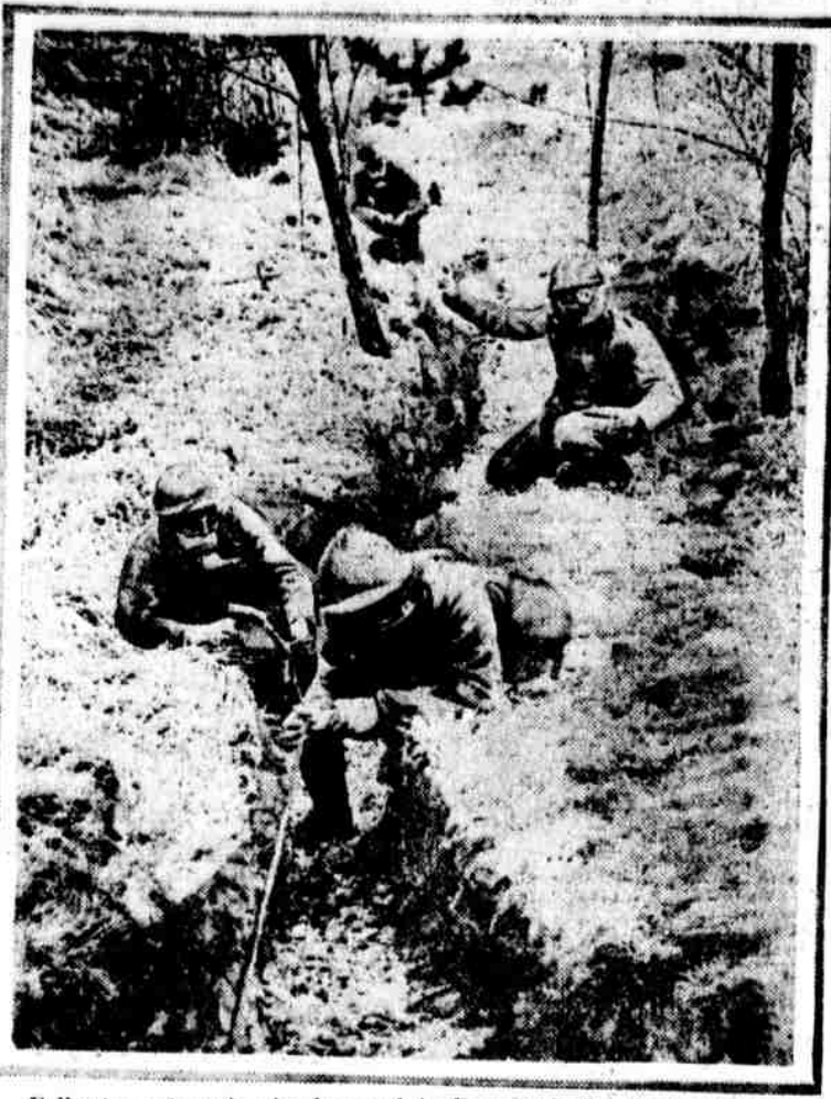
Following a fierce bombardment of the French trenches by the Germans, these French telephone engineers have been sent out to re-establish telephone communications, and are forced to wear gas masks while they work because of the German gas still lurking in the trenches
