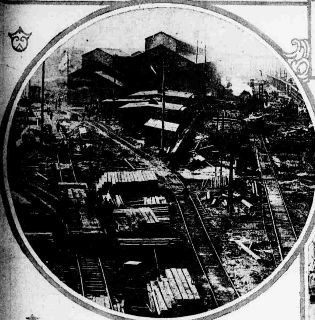
From the Eminence of One of the Giant Cranes the Shipyard Becomes a Beehive of Industry. In the Background Is the Original Plant of the Standard Cast Iron Pipe and Foundry Company, Which Was Purchased and Is Being Utilized by the Merchants' Shipbuilding Corporation.
