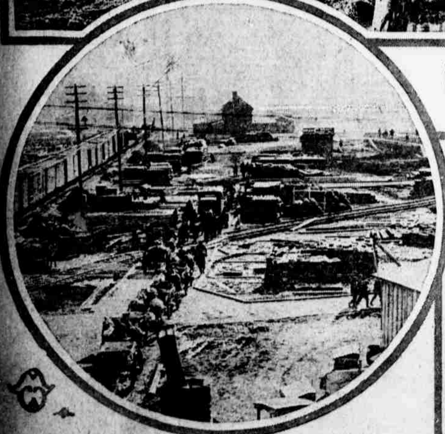
From a High Vantage Point at Twentieth Street and Oregon Avenue the Site of Uncle Sam's Great Shipping Depot Presents a Scene of Ceaseless Activity.
