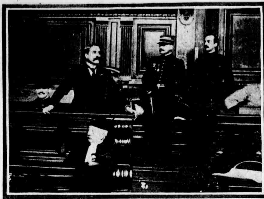
This is the first photograph to reach this country showing the trial of Bolo Pasha on the charge of treasonable intercourse with Germany, for which he was sentenced to death. Execution of this sentence has been postponed, awaiting the disposition of an appeal taken by the defense.
