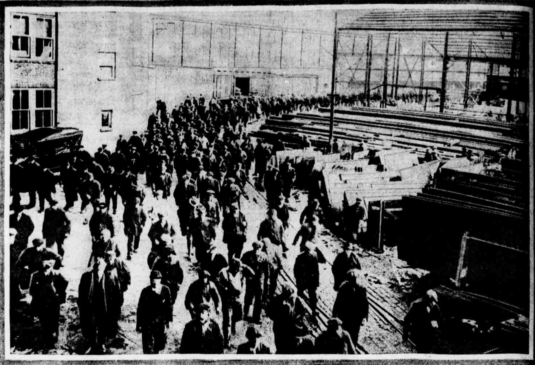
The Noon Hour at Cramps' Shipyards Permits of an Insight Into the Magnitude of the Shipbuilding Operations There, for it is Then That the Thousands of Workmen Lay Aside Their Tools and Pour Out of the Many Buildings for Lunch and a Brief Change of Scenery.
