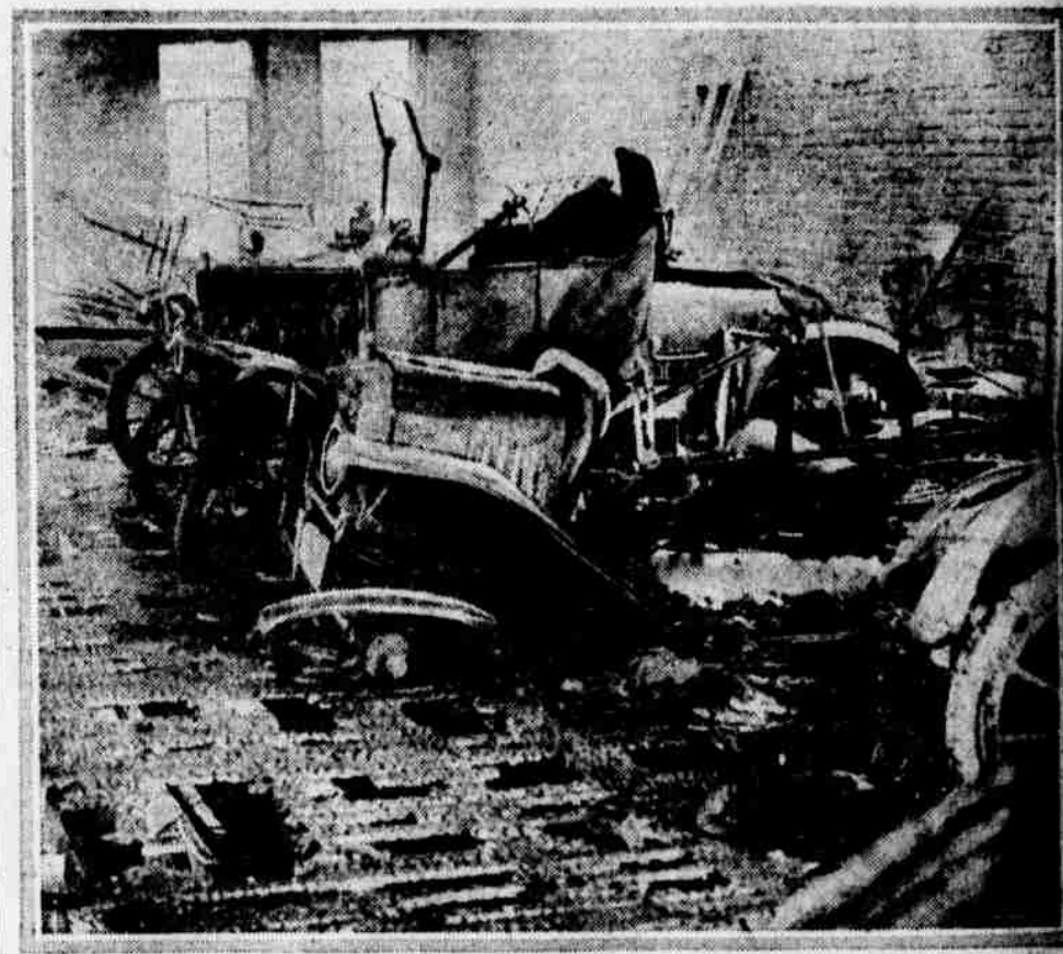
Scene in the Interior of the Ritner Garage, 1020 Ritner Street. After This Morning's Destructive Fire in Which Twenty-seven Automobiles and Nine Motorcycles Were Left a Tangled Mass of Debris.
