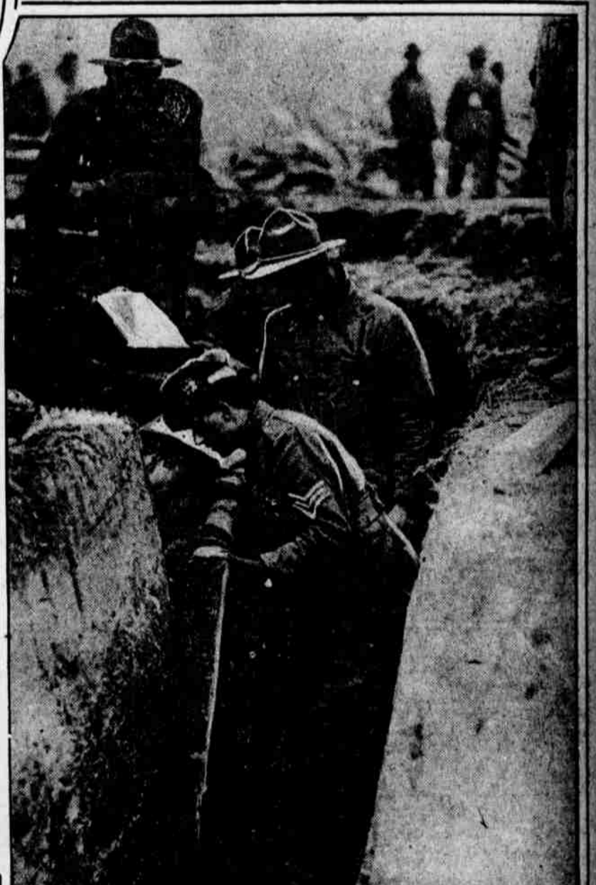
American soldiers in France mastering the details of trench construction with a veteran French soldier as instructor.
