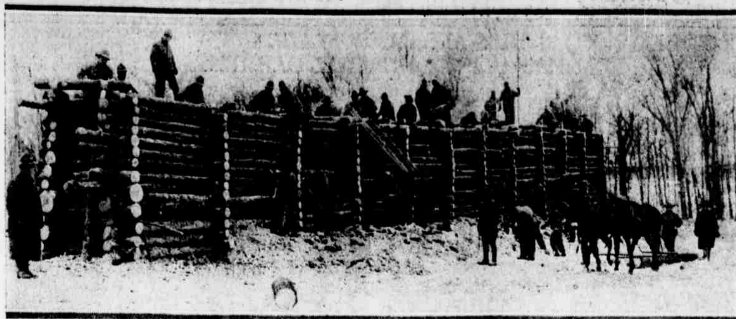
These soldiers are members of the 316th Regiment and have been pressed into service as carpenters for the erection of the stockade, which will be a part of the regiment's rifle range.
