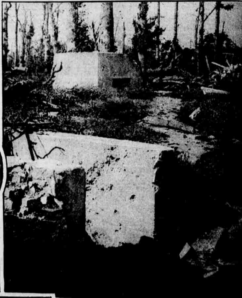
This Concrete Pillbox Represents Another German Trick When Failed to Refuel the British Artillerymen in France. It Was Erected in the Park Surrounding a Chateau, but Despite Its Clever Situation, Was Discovered and Shattered by British Gunners. In the Foreground Is the Entrance to the Pillbox. French Pictorial Press
