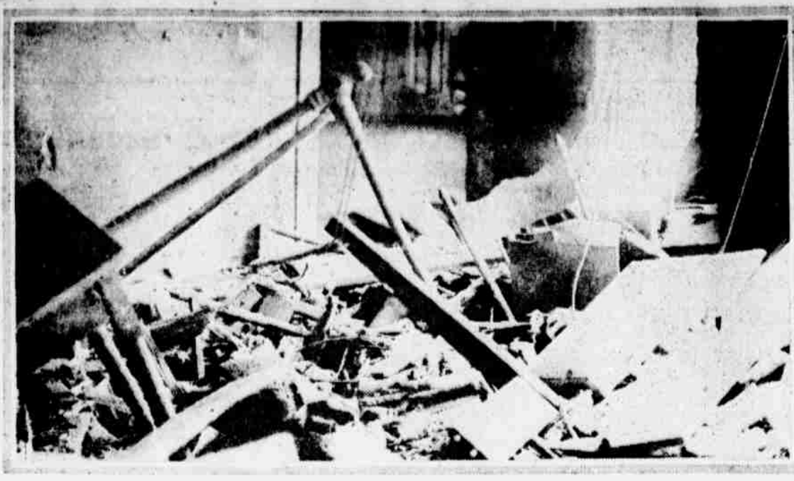
An explosion of the steam heater in the building at 1632 Walnut street this morning wrecked the three-story structure as completely as though it had been struck by a shell from a howitzer.
