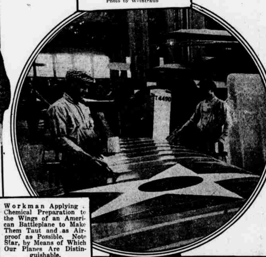
Workman Applying Chemical Preparation to the Wings of an American Battleplane to Make Them Taut and as Air-proof as Possible. Note Star, by Means of Which Our Planes Are Distinguishable. Committee on Public Information.
