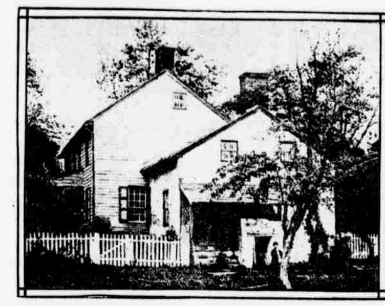
The modest buildings above at the left is the birthplace of Bayard Taylor; the other his home, Cedarcroft, which he built near Kennett Square.
