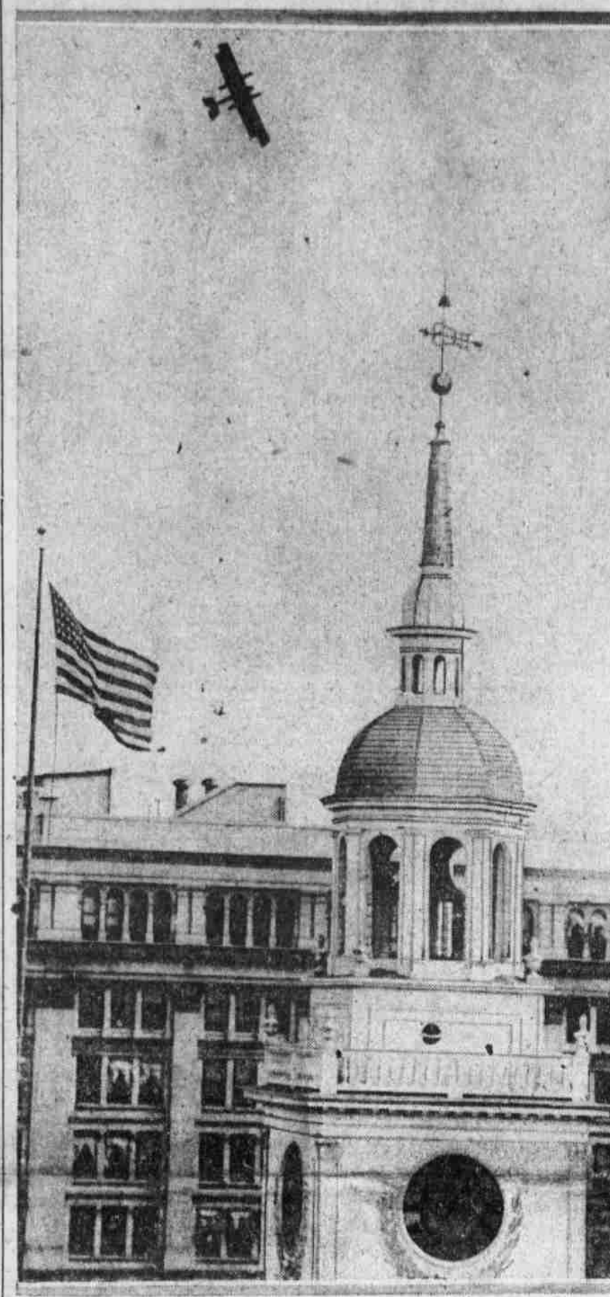
While the bell in Independence Hall steeps rang its iron-tongued call for subscribers to the second Liberty Loan today, airplanes in relays encircled the historic building, dropping circular invitations to citizens to do their bit by purchasing bonds.
