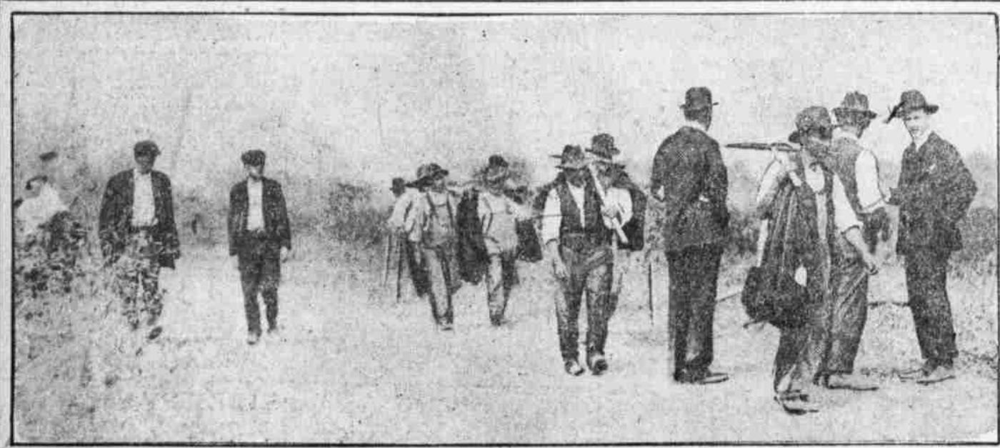
WORKMEN ON THEIR WAY TO WORK AT THE SITE OF THE PLANT
