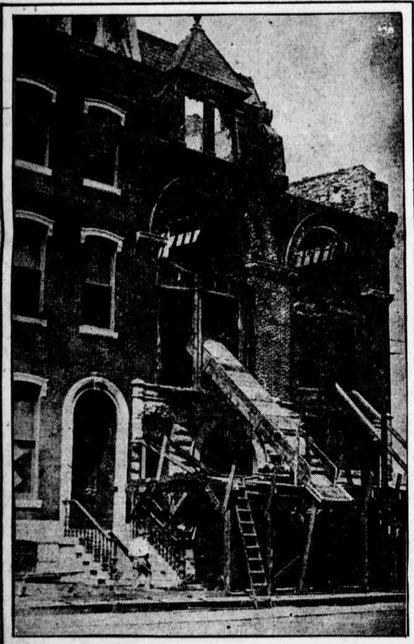
BEAUTIFUL RESIDENCES ON WEST SIDE OF LOGAN SQUARE GIVING WAY TO THE PARKWAY
