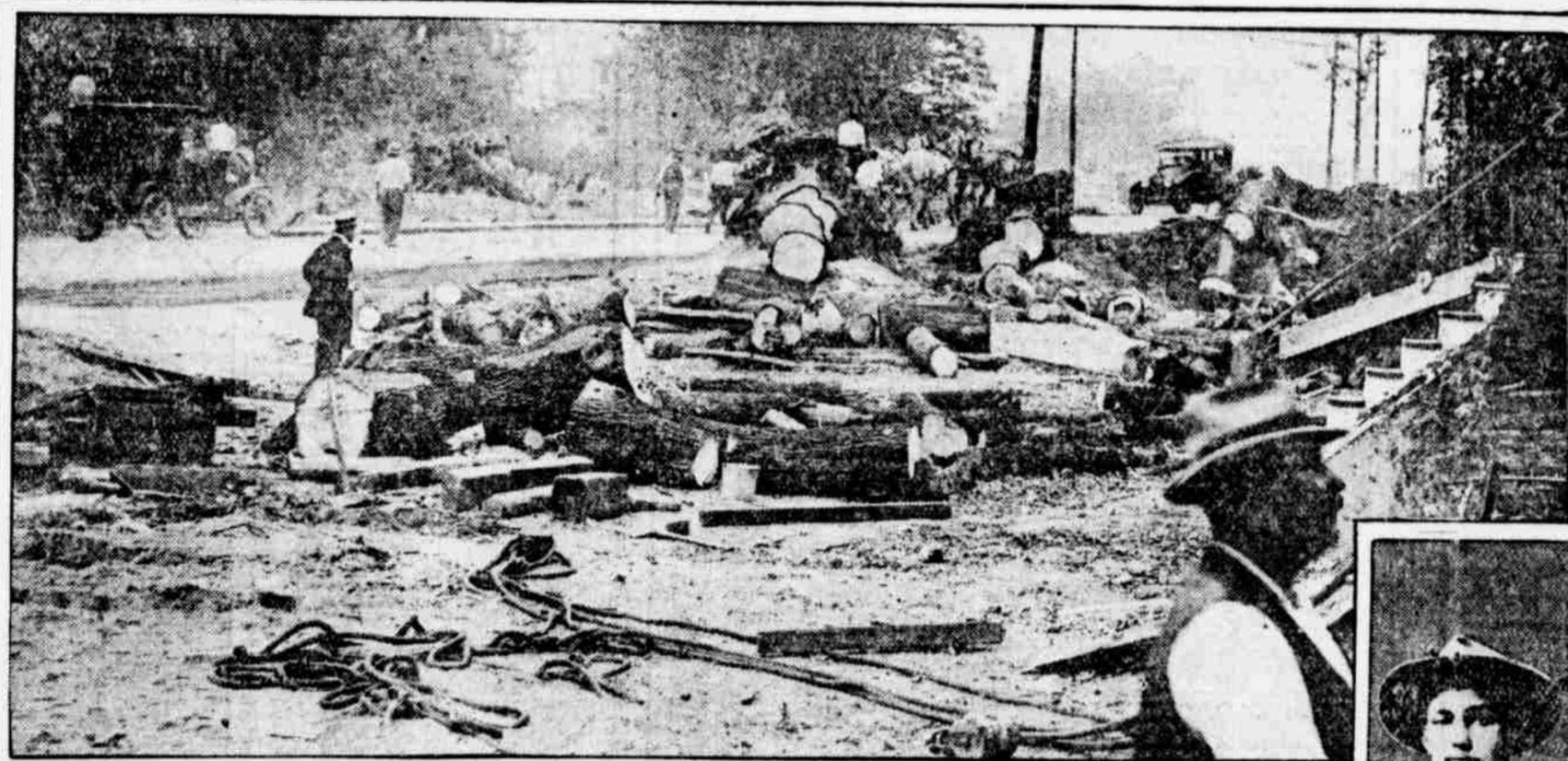
NO, THIS IS NOT A GLIMPSE OF A WESTERN LUMBER CAMP It is a metropolitan thoroughfare, being opened through Old York road beyond the Widener Home.
