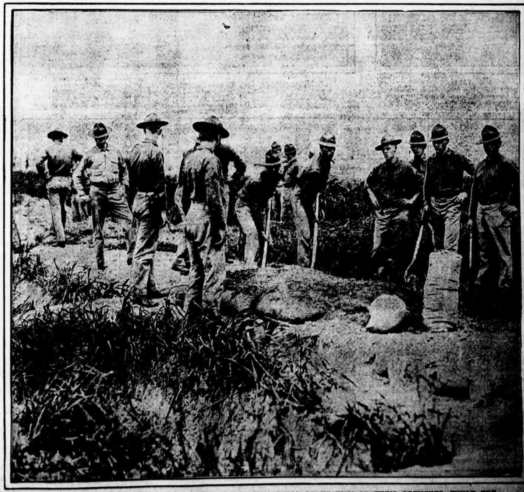
UNITED STATES MARINES PRACTICING TRENCH WARFARE OUTSIDE THE LEAGUE ISLAND NAVY YARD. THE MEN AT THE LEFT ARE LOADING SANDBAGS FOR PROTECTION OF THEIR TRENCHES, WHILE THE LARGE PHOTOGRAPH SHOWS THE TRENCHES BEING COVERED WITH EARTH TO FORM THE BREASTWORKS
